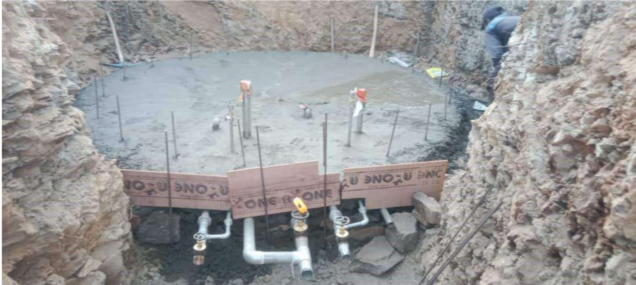
WASH systems strengthening and behaviour change in the hilly region of Makwanpur district in
